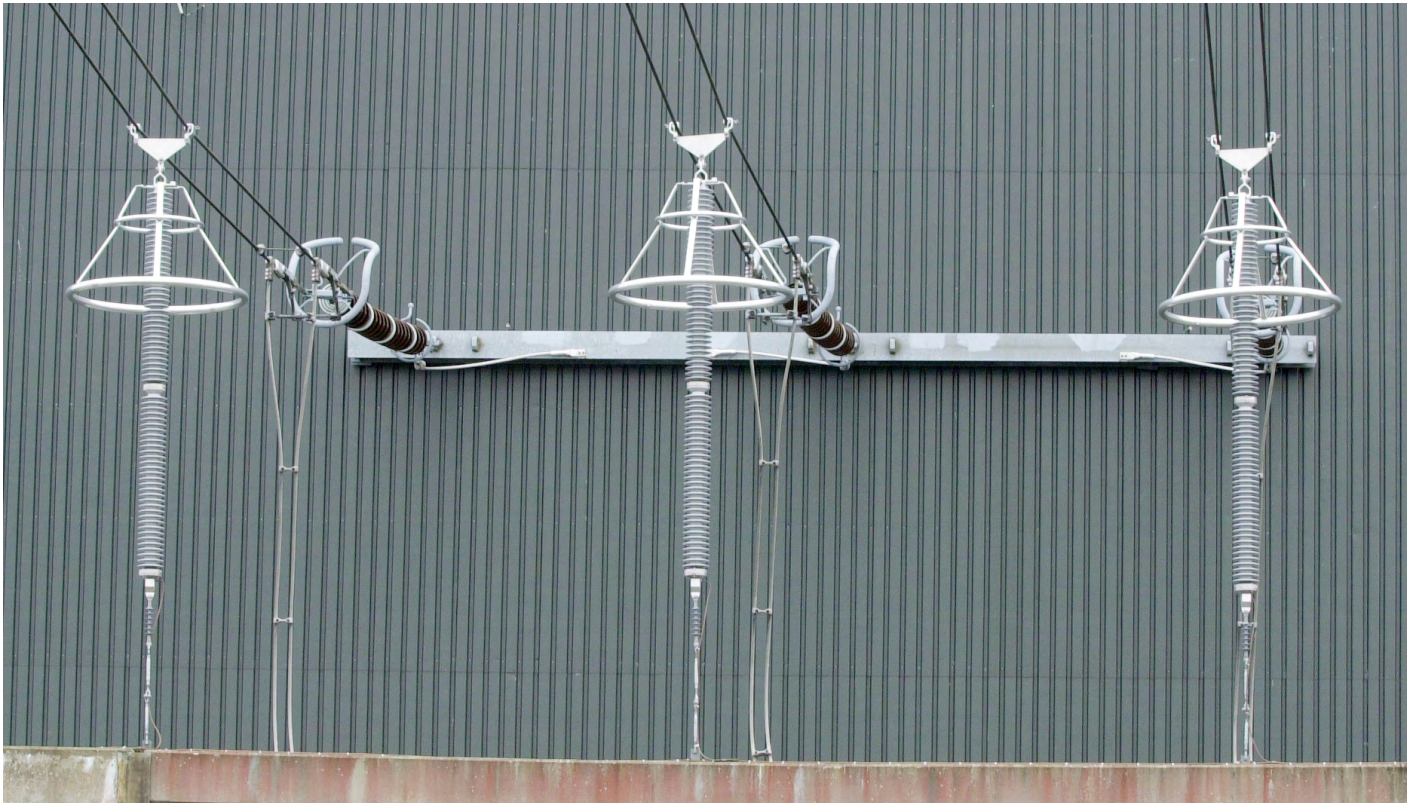
PEXLIM surge arresters connected to the 420 kV the secondary winding on a step-up transformer in a nuclear power plant
